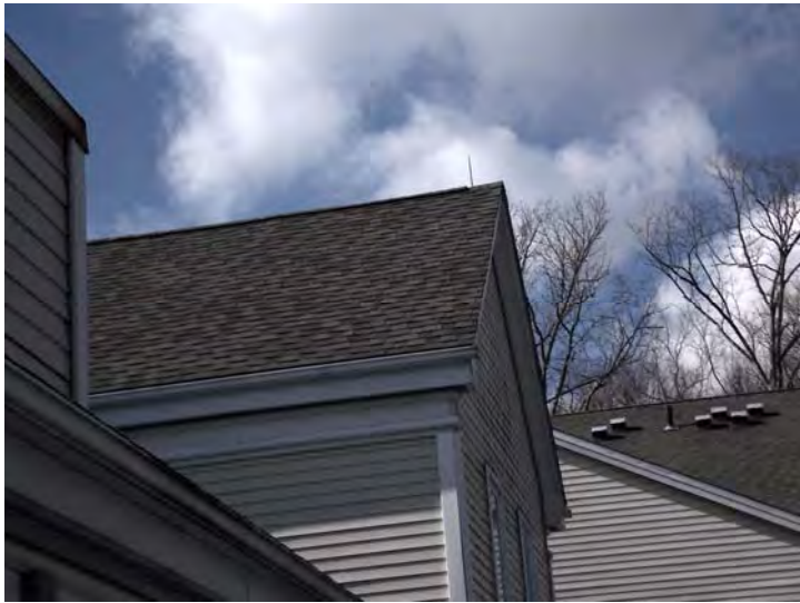
The roof is pitched and covered with architectural shingles.
