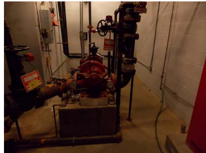
This is the firewater pump. It does not appear that a backflow preventer is in place (to keep stagnant sprinkler water from possibly contaminating the potable water).
