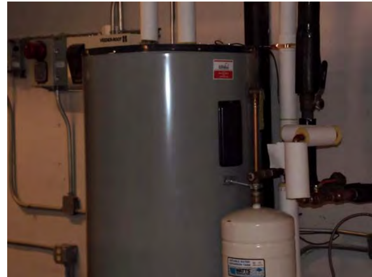
This is the DHW storage tank.
