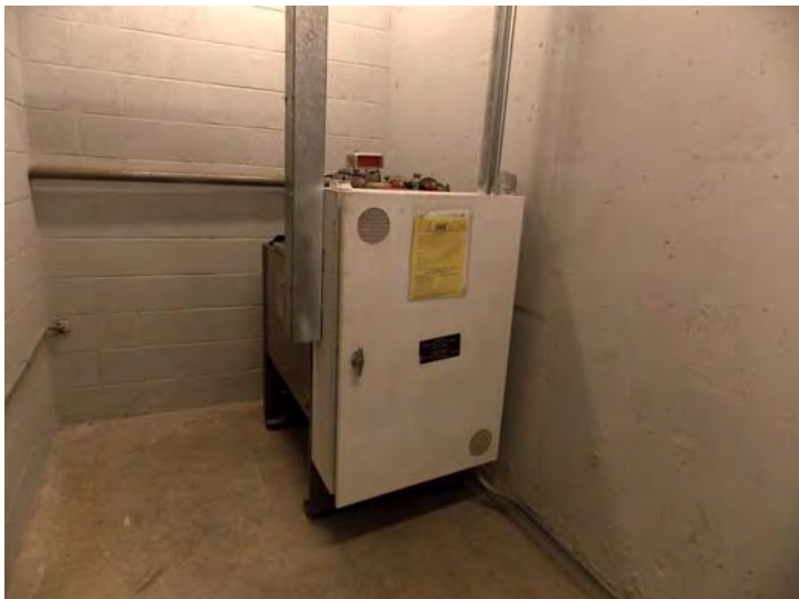
A view of the elevator's hydraulic pump station.
