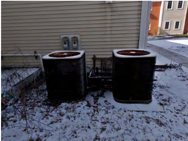
A pair of air-cooled condensers, part of two split DX air conditioning systems.
