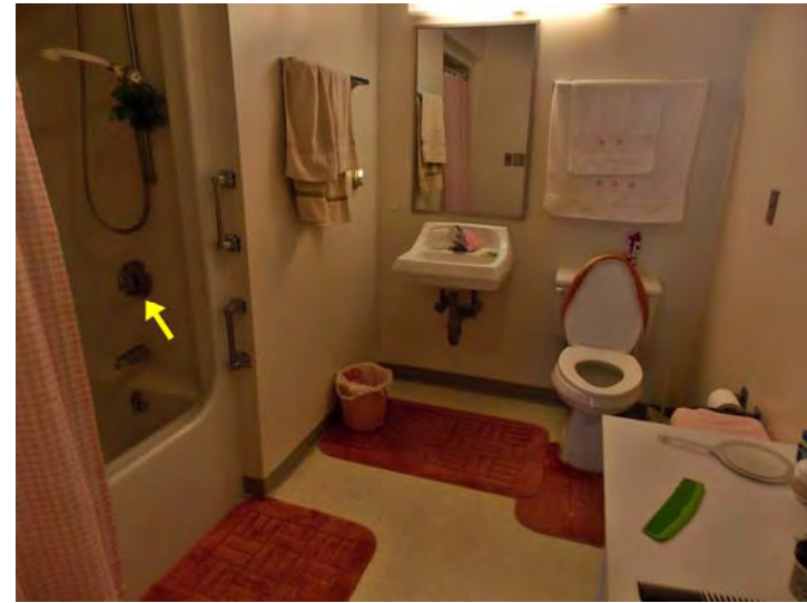
Bathrooms have wall-hung sinks and VCT flooring. The bathtub/shower includes an anti-scald mixing valve (arrow).
