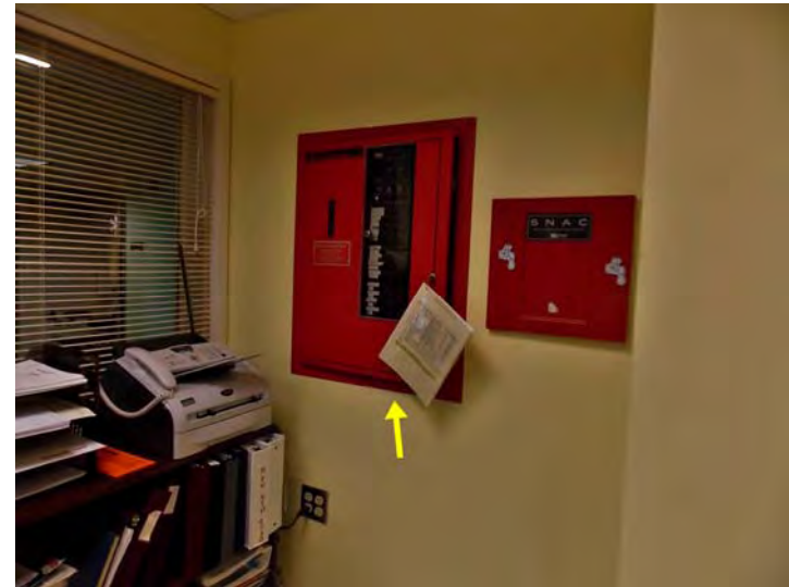
This is the central fire alarm control panel.
