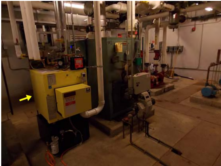
A view of the DHW boiler (arrow) and one of the hydronic heat boilers (green).
