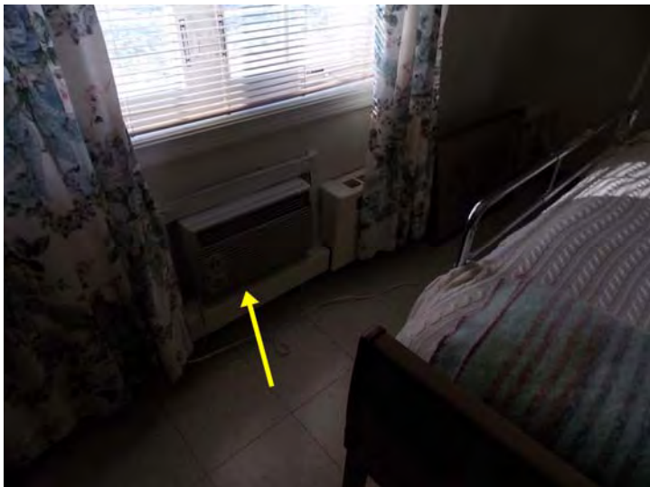
Through-wall sleeves are provided for unit air conditioners.
