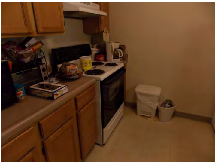
Kitchens have wood cabinets, laminated particleboard countertops, electric ranges, and VCT flooring.
