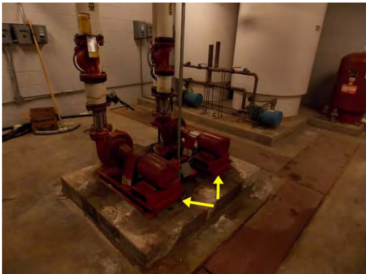
These are the hydronic circulating pump. In the background are the well-water pumps and storage tanks, no longer in use.
