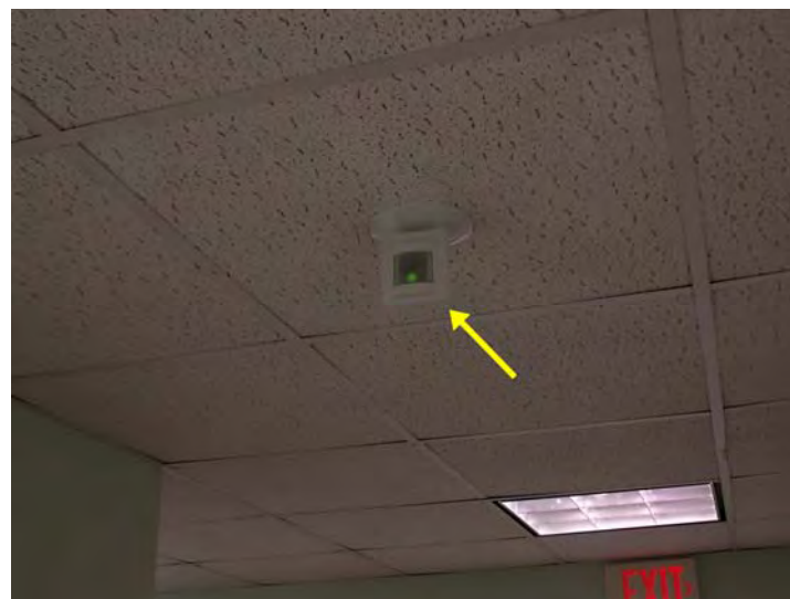
Occupancy sensors are used in the common hallways to control the lighting. During unoccupied periods, 50% of the lights will be turned off; once someone is in the hallway, all of the lights are turned on.
