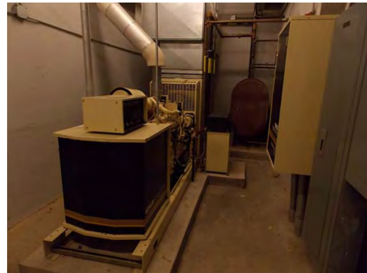
This diesel-powered generator produces 100 kW of emergency power.
